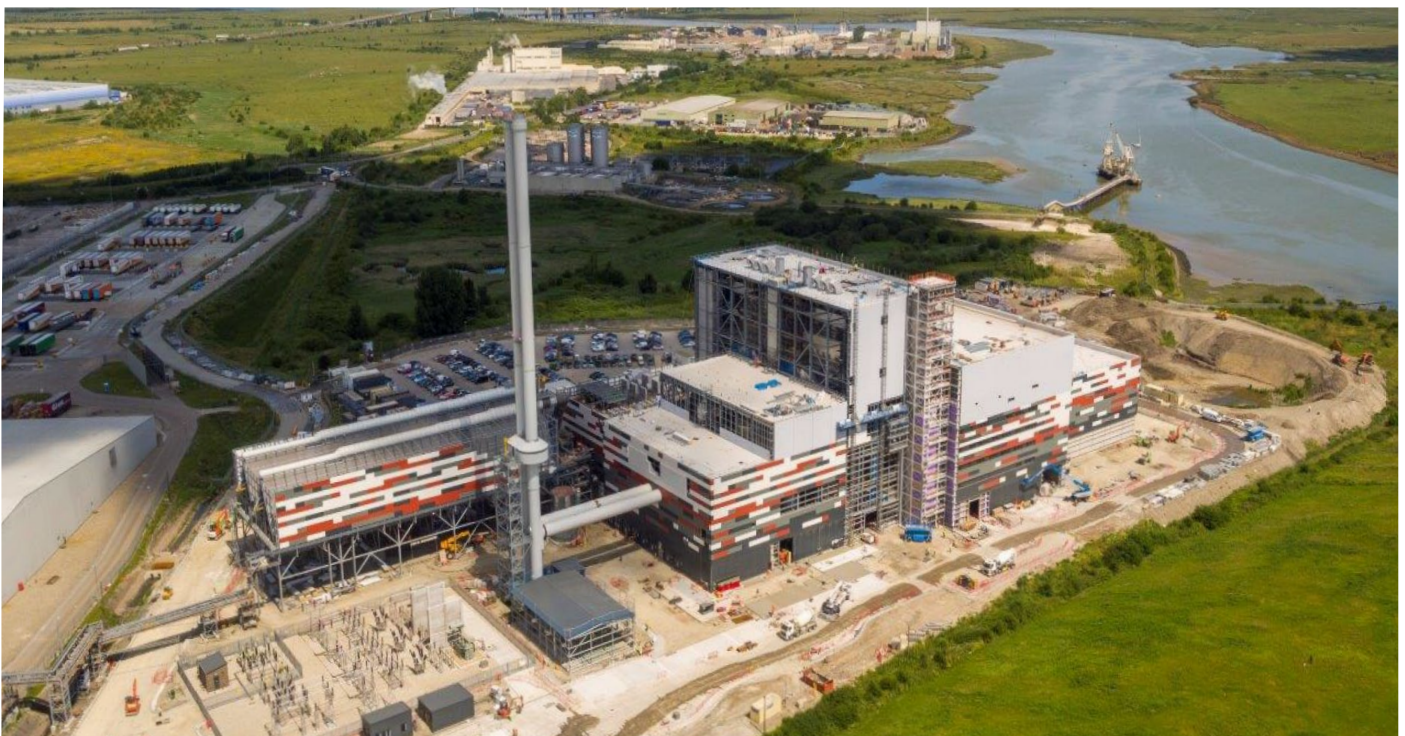
Figure 3: Photograph of the K3 facility under construction in July 2019.
